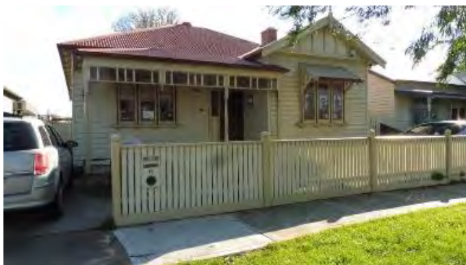
Hipped-roof weatherboard bungalow with corrugated iron roof, red brick chimney, vertical strapping and finial, timber-framed casement windows with leadlights, window canopy with fretted brackets, exposed roof rafters, verandah under roofline with timber frieze at 6 Stanley Street. Source, M. Summerton, 2020
