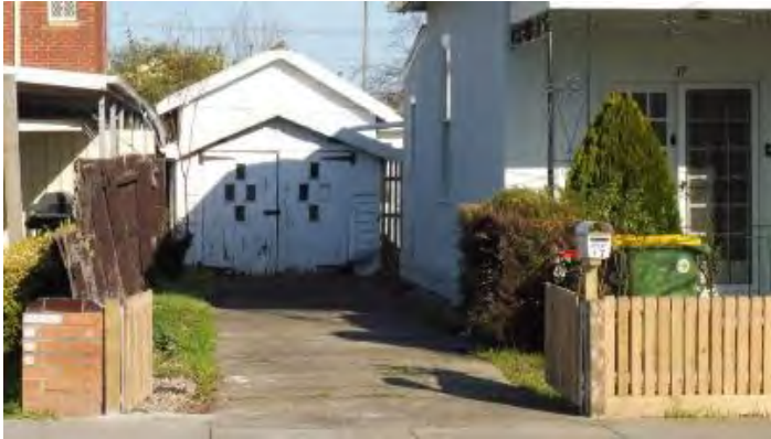
Original hinged timber garage doors with patterned glazing at 17 Wallace Street. Source, M. Summerton, 2020
