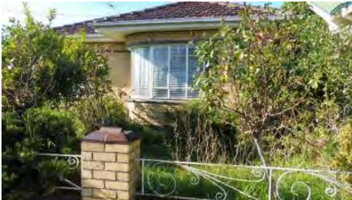
Post-war cream brick veneer with 'waterfall front'. Robin Boyd [1952, p100], uses this stylistic term and writes 'The more pretentious house of the World War II period was given rounded corners – a streamlined effect'. Manganese brick detail, steel casement windows, glazed roof tiles and wrought ironwork also typify the style. 15 Stanley Street. Source, M. Summerton, 2020
