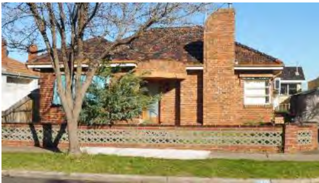
Double-fronted clinker brick veneer bungalow with glazed terracotta tiles, curved porch parapet, curved chimney, steel-framed windows, and matching fence with concrete breeze block panel at 49 Napoleon Street. Source, M. Summerton, 2020
