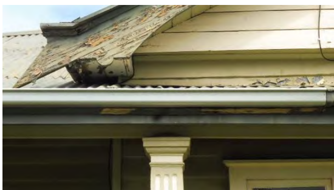
51 Hansen Street. Detail of original decorative timber bargeboard end to the front gable. Source, M. Summerton, 2020
