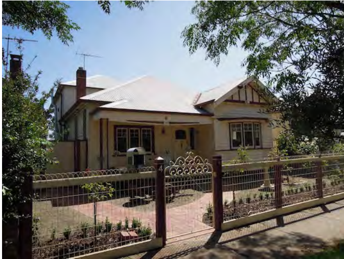
Naismith Street, Showing typical roof form with hipped roof, extending to form lower hipped roof over the front verandah, projecting gabled section, with bracketed gable end, and bow window. The unusual verandah roof beam detail tapering to the ends with cut out decoration is typical of the houses on the north side. Twisted wire fence not original but appropriate. Rear two storey addition. Source, M. Kenna 2020
