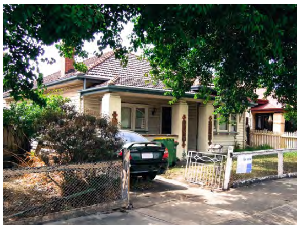
13 Summerhill Road, Footscray, typical of the Inter-war houses of the precinct and likely to be built by A.S Whitehill, with terracotta tiled hipped roof, round-edged weatherboards, rendered square brick columns to verandah with tapestry brick details, original timber-
