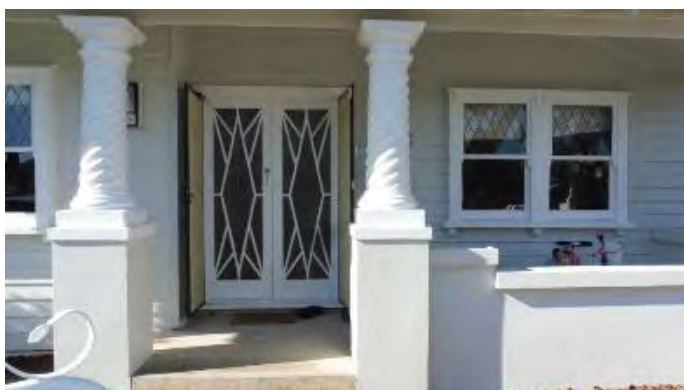
17 Stanley Street. Weatherboard Californian Bungalow with timber framed, glazed double front doors and windows with diamond lead lights in upper sashes. The barley twist columns flanking the verandah step are an example of the Revivalist styles which influenced late 1930s bungalow designs. Source, M. Summerton, 2020
