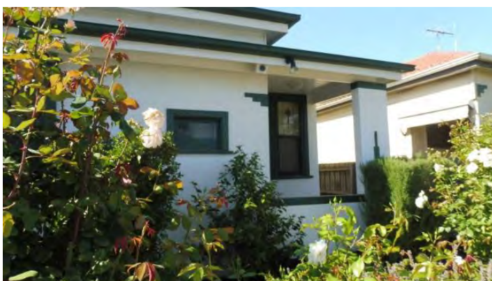
Numbers 1A and 2A Nesnah Street are atypical of houses in the Hansen Estate. They were built on narrower allotments at the end of the dead-end street, with no provision for side drives. The freestanding pair share basic, functional forms with conic facades, small enclosed porches, and windows with decorative lead lighting. 1A retains its original roof of metal, simulated terracotta tile sheeting. Source, M. Summerton, 2020
