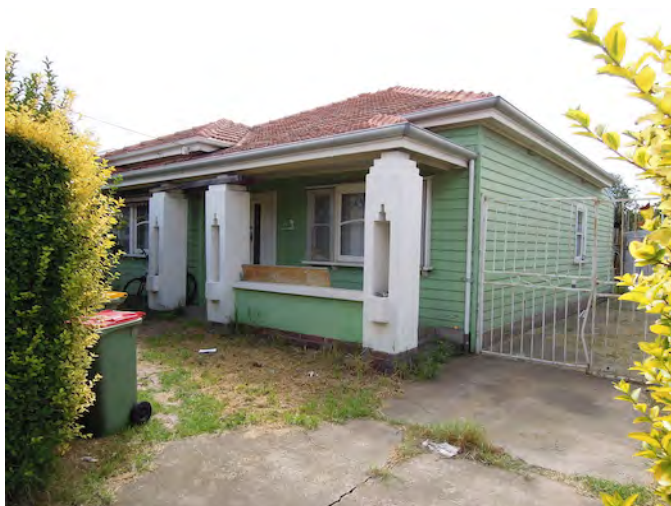
13 Dempster St, West Footscray. The houses in Dempster Street were completed before those in Fontein, Gwelo and Sredna Sts and have features more typical of the later Inter-war period-decorative piers supporting the verandah roof have niches and tapered tops. Timber framed windows have decorative leadlight to upper sashes. Source, M. Kenna, 2020
