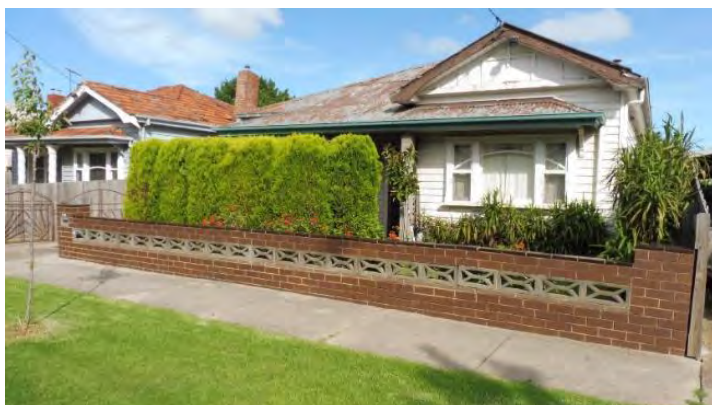
25 Hansen Street. Brick and concrete breeze block fence built in the 1960s, and wrought iron gates. The fence fabric is inconsistent with the period but the scale is acceptable. Source, M. Summerton, 2020
