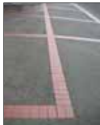
indicative paving banding asphalt with brick pavers, in a rectangular or lineal pattern.
