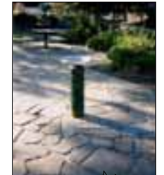
focus areas fractured bluestone or charcoal concrete to 25Mpa with random trowelled groove expressed.
